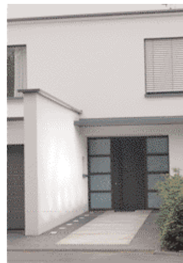
The guide wall at the entrance receives soft light from a series of diffuse inground luminaires. The line of luminaires underscores the path to the front door.
