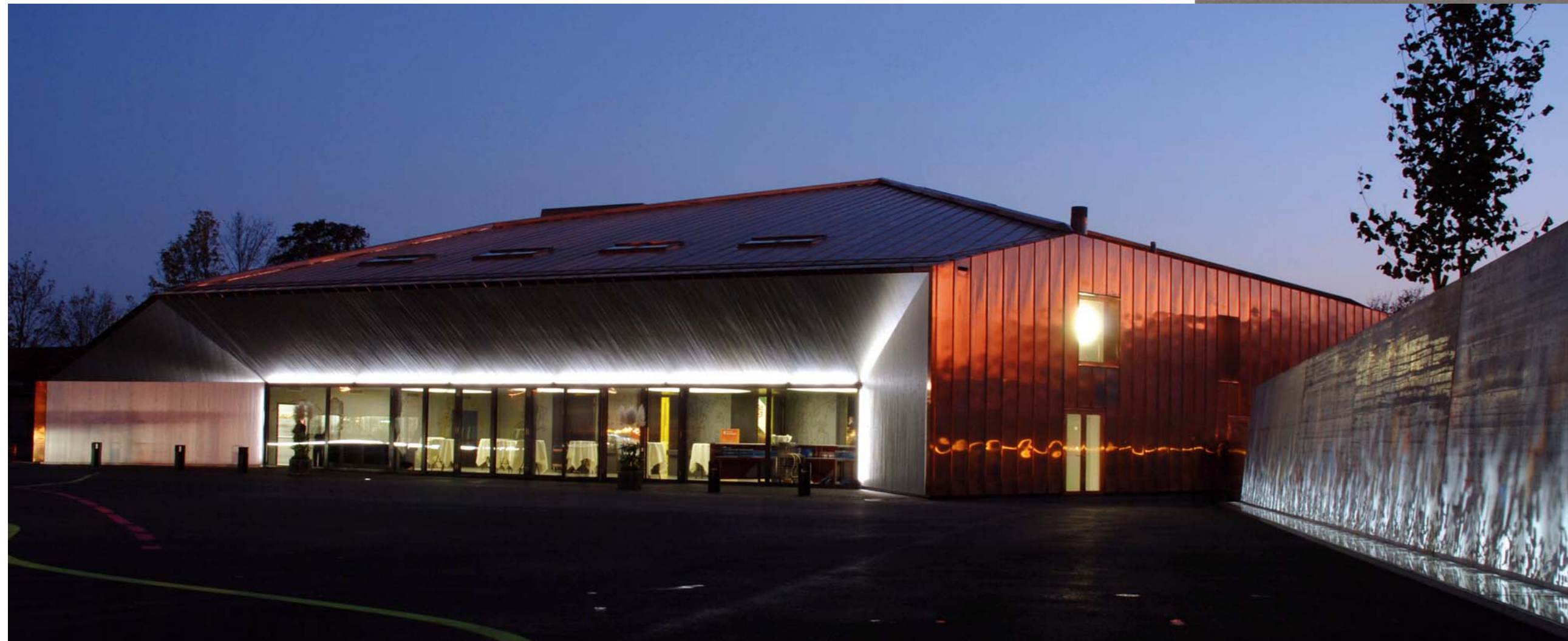
Left: Square showing the festival hall from the front: in spite of the fact that the hall can accommodate up to 2500 people, the building remains reticent in volume, its dimensions blending in with the scale of the existing environment. The festival hall itself is closed on three sides, which supports its marquis character. The festival hall façade opens up in the form of a huge portal, drawing visitors in through the funnel-like entrance. This effect is further enhanced after dark by the lighting, which outlines the almost archaic portal on three sides in harsh white light.
